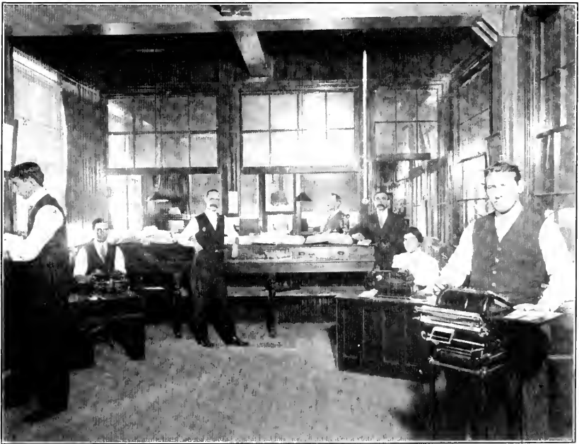
BUSINESS AND PRIVATE OFFICES OF THE WOODBINE CHILDREN'S CLOTHING CO.
